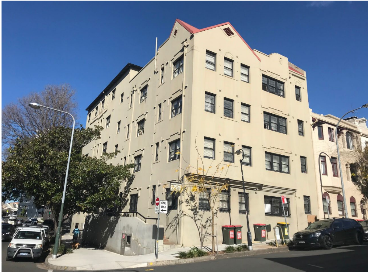
adjoining building to the north, fronting Kellett Street
